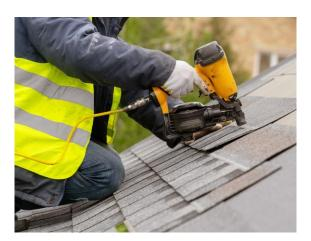
Pneumatic tools must be checked to ensure the tool is fastened securely to the air hose.
